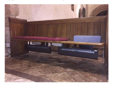
Another option is to sue fabric covered Cooltouch heaters as below, which appear to be available in longer lengths so only 26 would be required.
