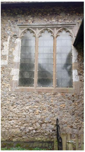
The windows are noted to be protected by plastic (probably polycarbonate) sheeting on the outside. This is not airtight, but measurements at other churches have shown that it does prevent heat loss with the glass no longer being the coldest surface. The PCC should note that polycarbonate panels will not last forever, they tend to yellow with age and become brittle. The "bulletproof" quality only applies when new as they suffer from degradation under UV light.
