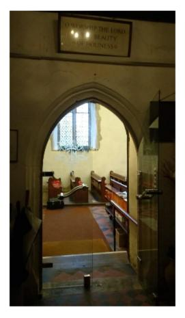
Where a timber door closes against a timber frame it is recommended that draught proofing is fitted. A product called QuattroSeal (see link below) is often used in heritage environments to provide appropriate draught proofing.
